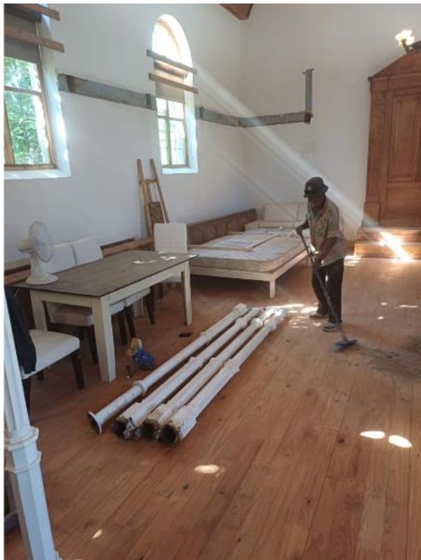
Renovations in progress
